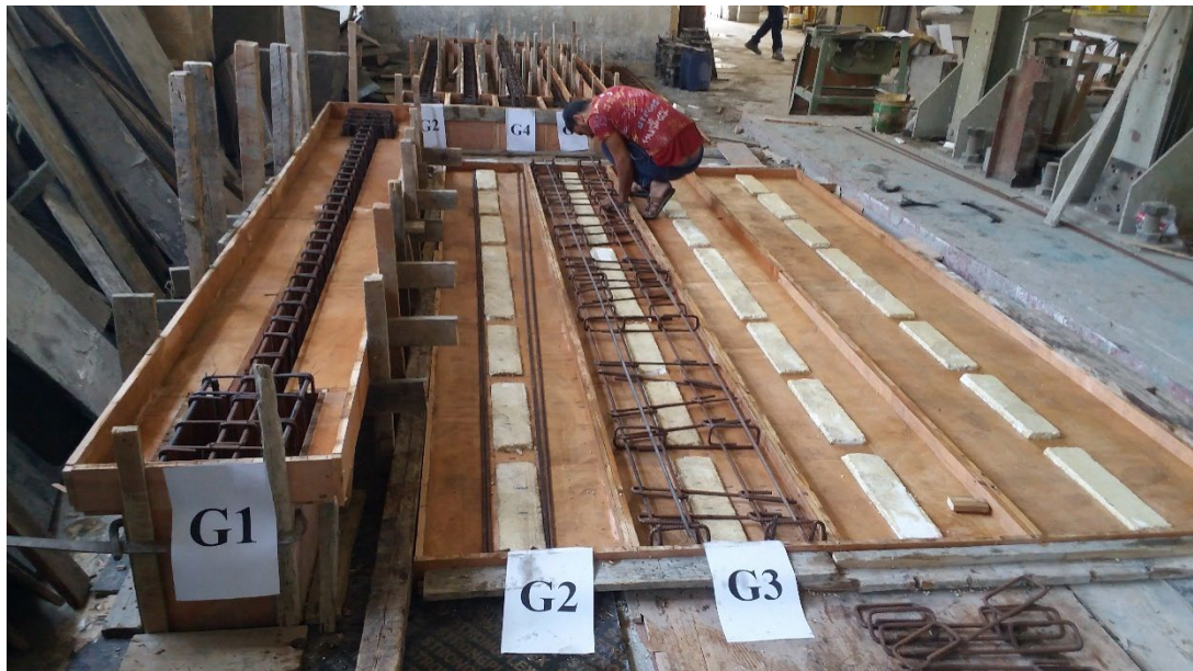
Figure 8: Preparation of reinforcement for tested specimens
