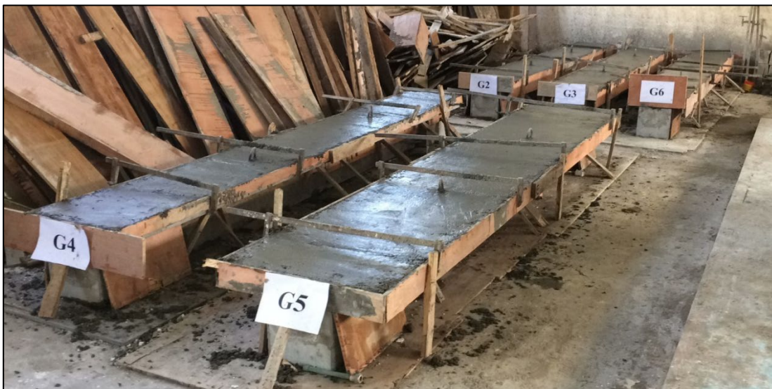
Figure 15: Finishing casting concrete for the rest of topping slab (G2 to G6)
