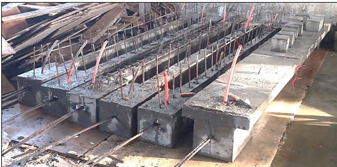
Figure 10: Control specimen G1 and five girder webs
